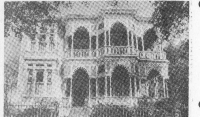
QUEEN CITY OF THE SOUTH... Galveston, Texas, is nationally known for its Victorian architecture. Shown is the famous Sonnenthil House built in 1886.
