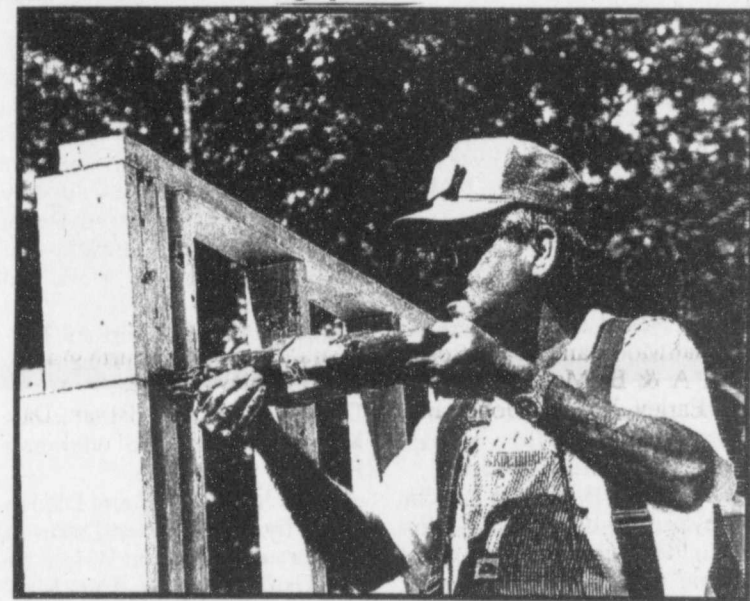
EDDY DENNY , member of the First Baptist Church of Bogata, works on a Texas Baptist Men Retiree Builders construction project near Paris, building a home for an 11 year old girl and her family.
