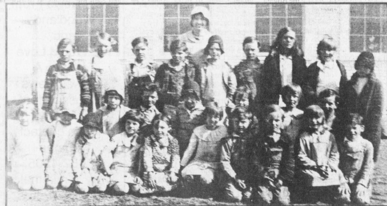
LINE BRANCH SCHOOL located between Bogata and Clarksville in 1927 is the date this photo was taken. We know somewhere in the photo are V.A. Crump, Lela Crump Brown, Lessie Crump Parker. The photo was brought in by Frances Mathews of San Angelo. If anyone knows the identity of the others in the photo, please call 652-4205 or 632-5322.
