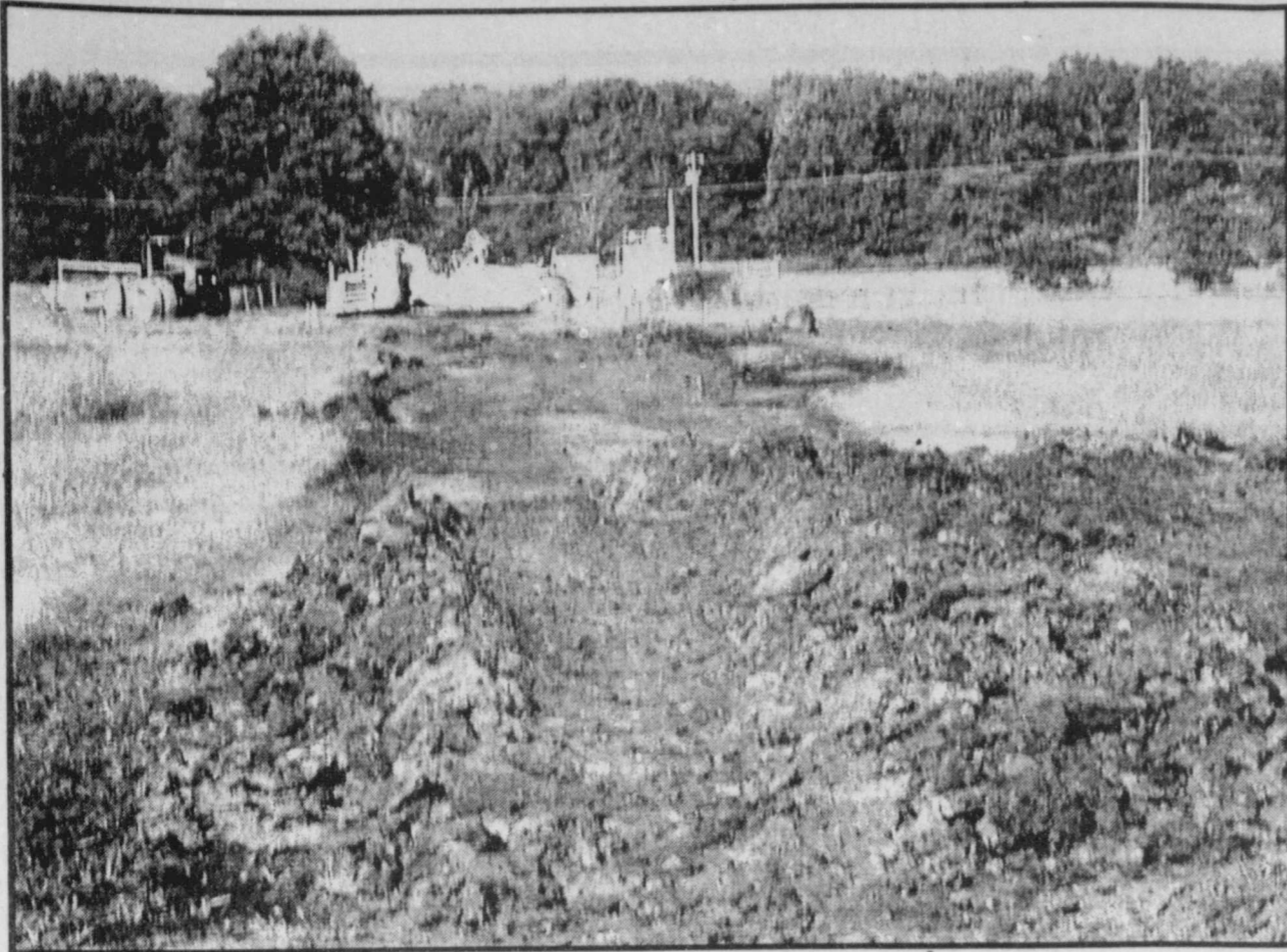
DELAYED-The dirt work which was to have been started at Rivercrest has been rain delayed. Although machinery attempted to begin progress recent rains put a quick halt to the work. (Staff Photo Nancy Brown)
