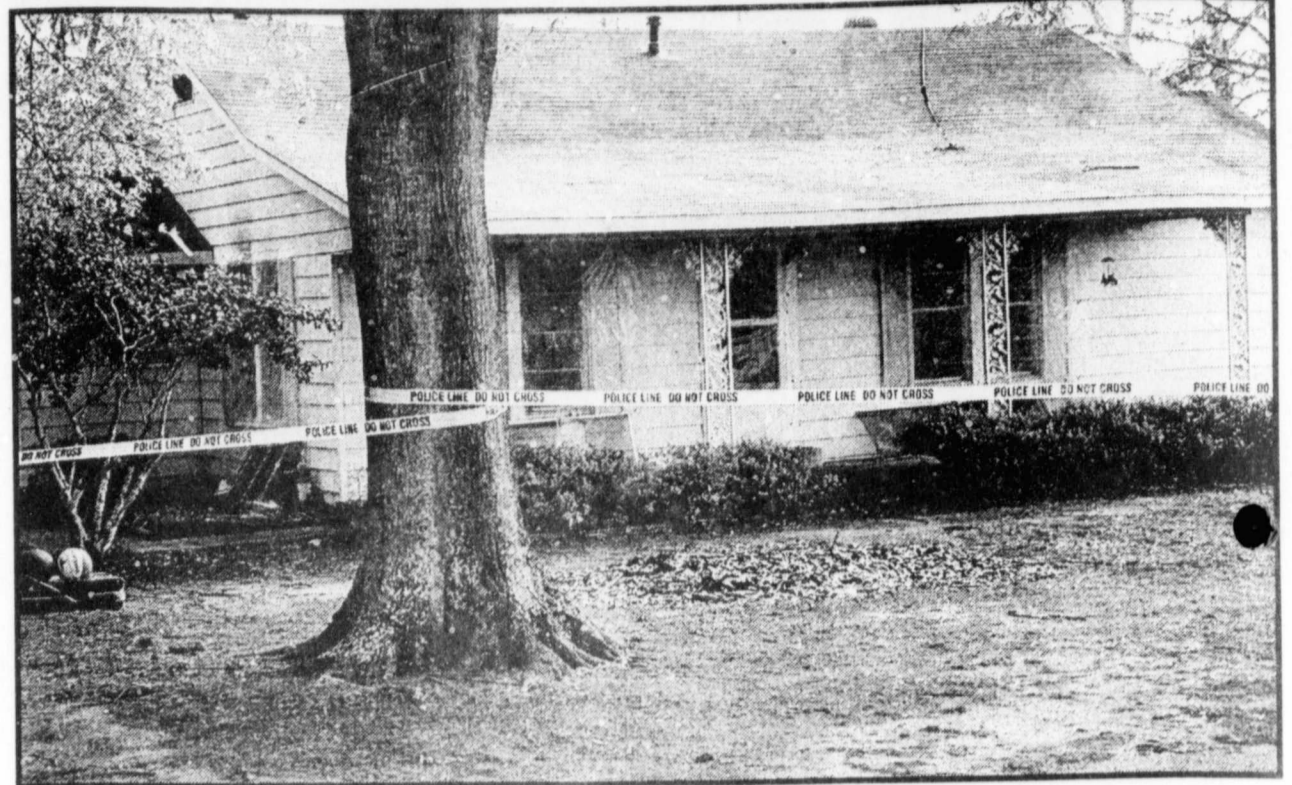
GUTTED —the house, belonging to Kelley and Deana Boyd of Bogata suffered heavy damage from fire Friday night. Bogata Volunteer Fire Department was on hand to fight the blaze. (Staff Photo by Nancy Brown)
