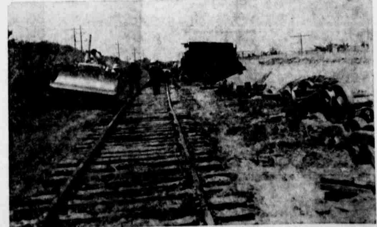
TRAIN CARS DERAILED—Four boxcar loads of wheat were thrown off the track, between Rule and Rochester over the weekend. Cause may have been due to recent high water along the right-of-way after rains up to 16 inches fell in that part part of the county. (Staff Photo)
