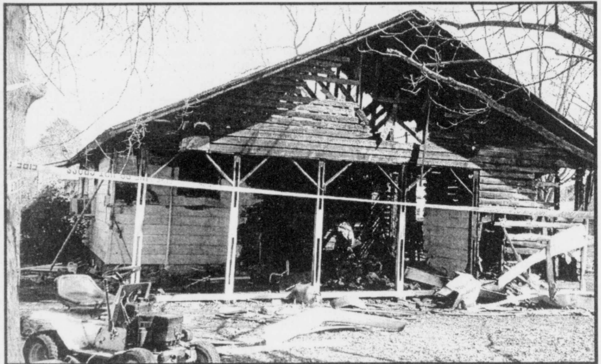
THE HOME OF BOBBY AND DENA LUTTRELL of Bogata was gutted by fire on Sunday, March 14 in the early hours of the morning. The cause of the fire was possibly electrical. (Staff Photo by Judy Screws)
