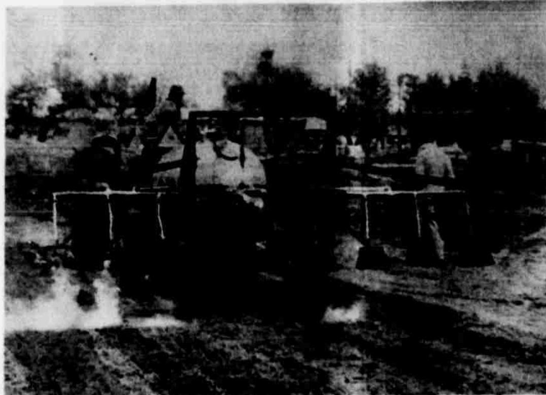
COOKING WITH GAS . . . When it gets too wet for a tractor pull you simply heat the ground until all moisture is evaporated, pack the dry dirt and proceed. Sound simple? If you saw the condition of the ground last Saturday before work began you wouldn't think so. Many hours of labor were necessary before the track was finally complete. Almost 1,000 gallons of butane were used in drying the ground. This burner and 500 gallons of butane were donated by Penman Butane of Rochester. Haskell Butane donated 500 gallons of butane to help make the event possible. Staff Photo by D. Comedy.
