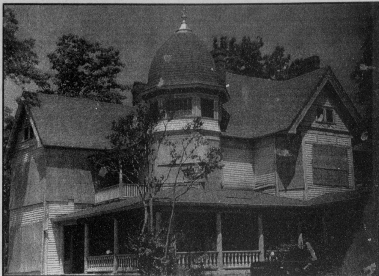
WORK IN PROGRESS -The Red River County Historical Society is in the process of restoring the Lennex home in Clarksville. According to the Historical Society President Jack Herrington the project is expected to be completed by the end of the year. President Herrington purposes the house be used for special occasions such as service clubs, weddings and etc.
