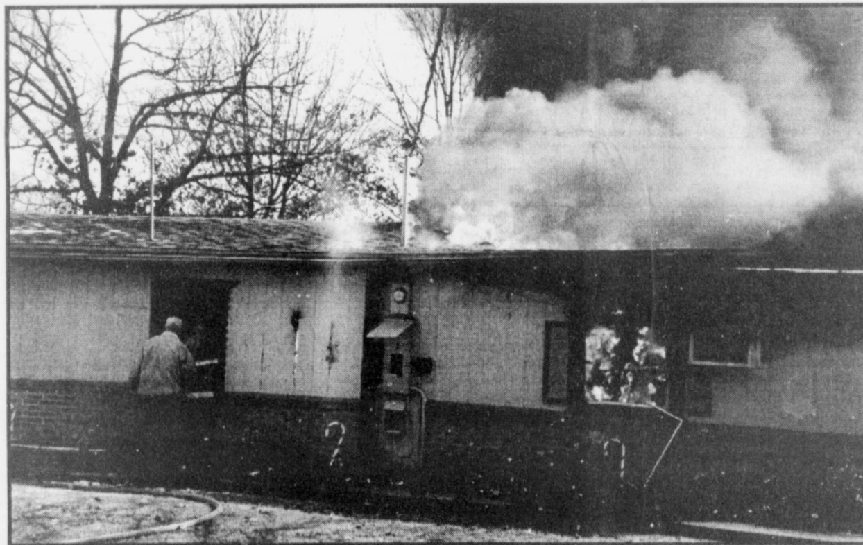
FIRE ENGULFED Global Genetic Engineering Labs facilities on Highway 37 south of
