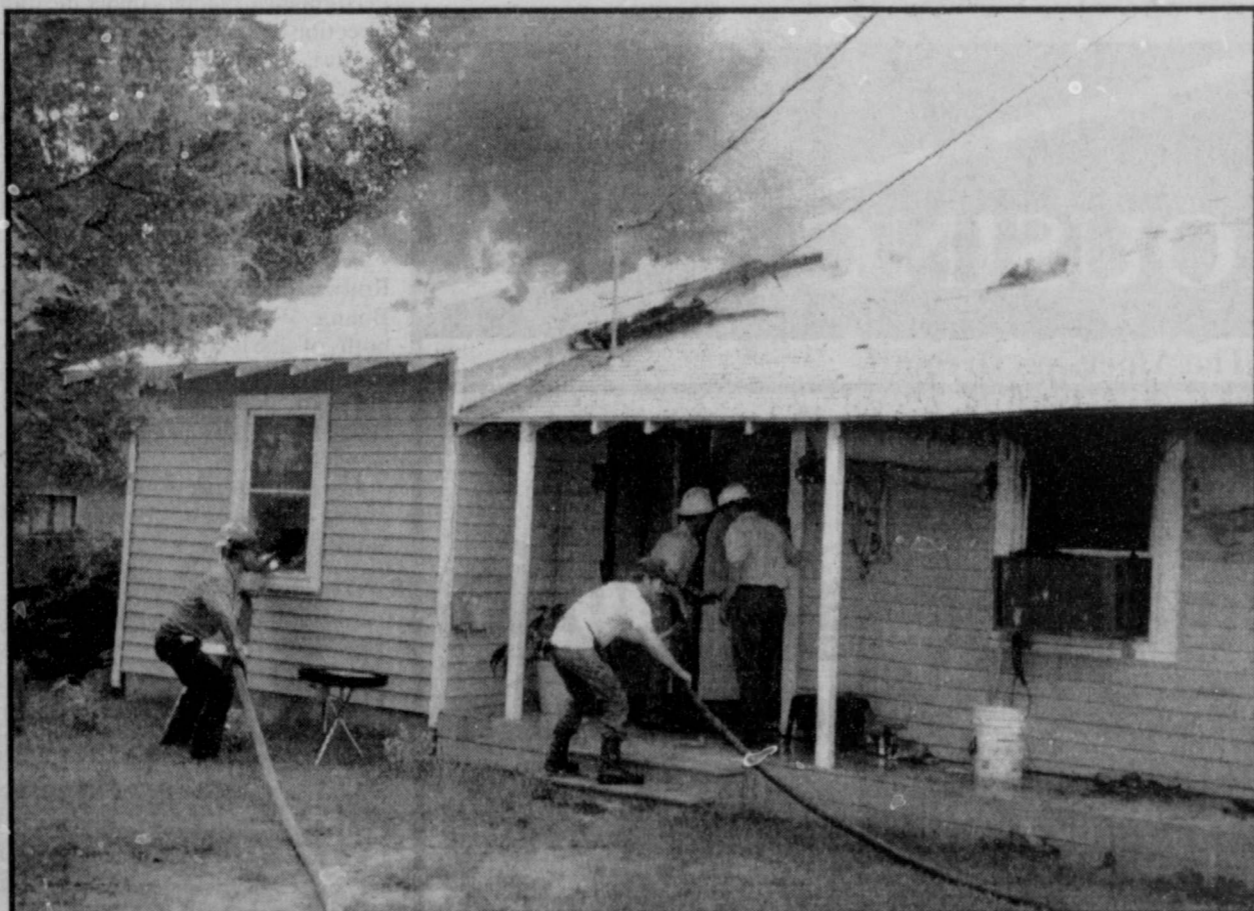
BURNING-Bogata Volunteer Fire Department responded to this house fire on South Main Tuesday afternoon. The house belongs to the Ronny Merchants, who were not at home at the time. Lightning is thought to have struck the building, which suffered heavy damage. (Staff Photo by Judy Screws)
