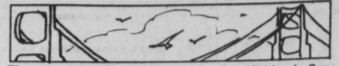
The two main cables on the Golden Gate Bridge in San Francisco hold 80,000 miles of wire.
