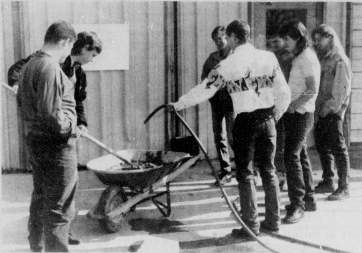
MIXING CONCRETE for work on the meat lab at Rivercrest
