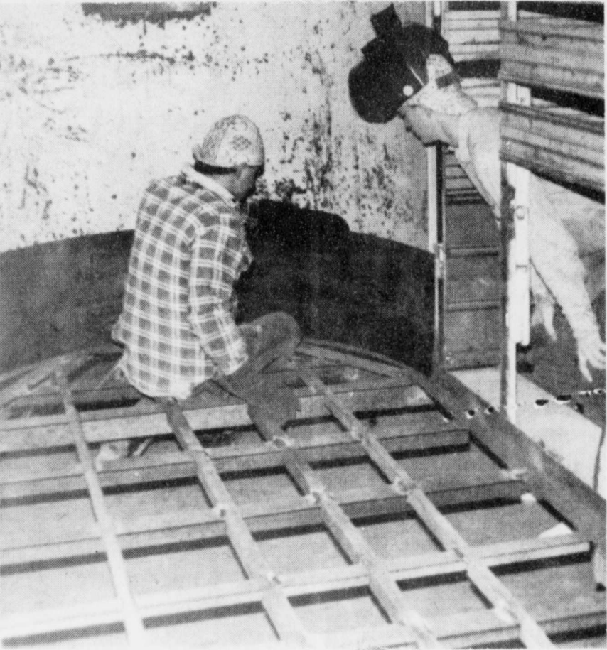
NEW FLOOR-James Hampton and Scott Yancey, both members of the Rivercrest FFA Chapter, install a new metal
