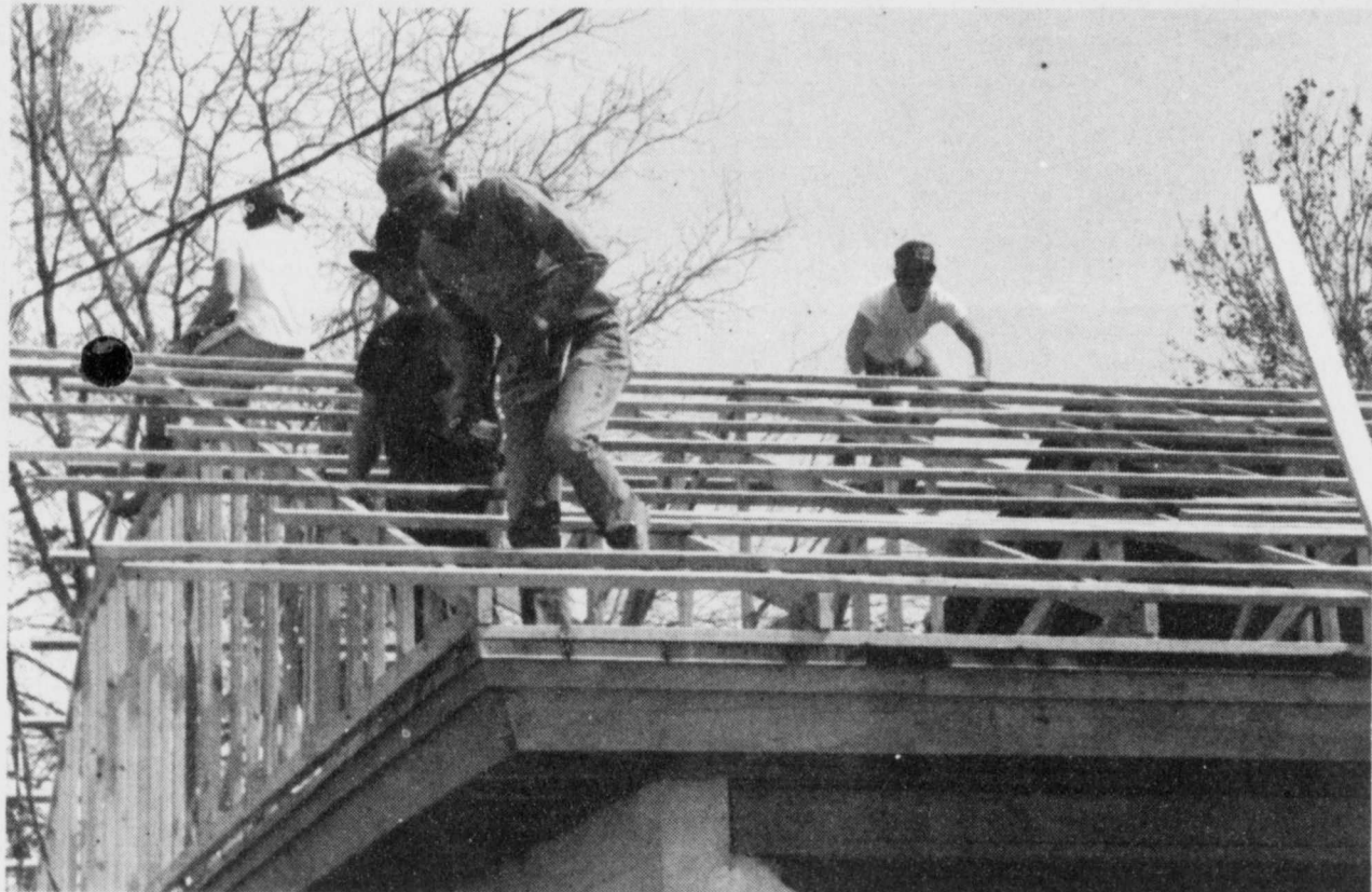
BOGATA VOLUNTEER Firemen put a new roof on the fire station
