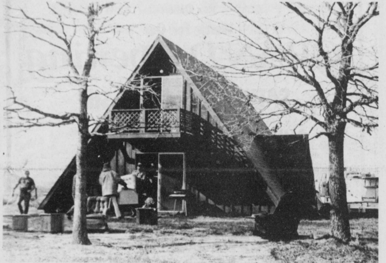
HEAVY DAMAGE -The home of Don and Judy Screws, located on Hwy 271 just out of Bogata, was
