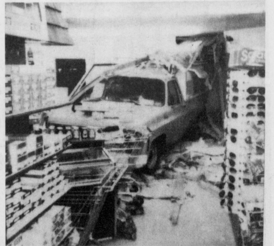
UNAUTHORIZED ENTRY! This pickup, driven by Jerry Knight of Bogata, crashed through the north wall of Dean Ward's Grocery
