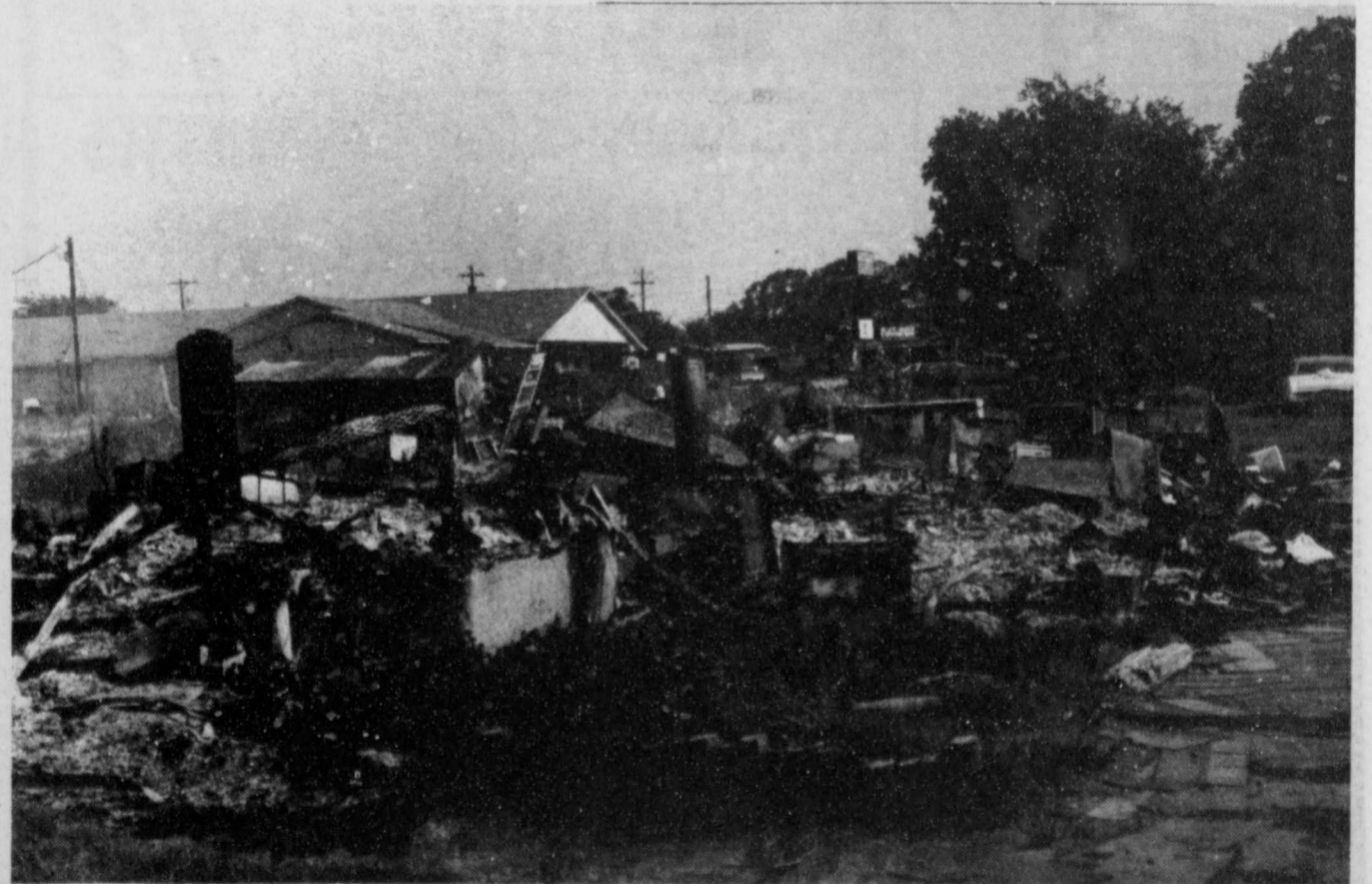
DESTROYED—The Bobby Martin home in Bogata at 2nd St. S.W. was destroyed by fire
