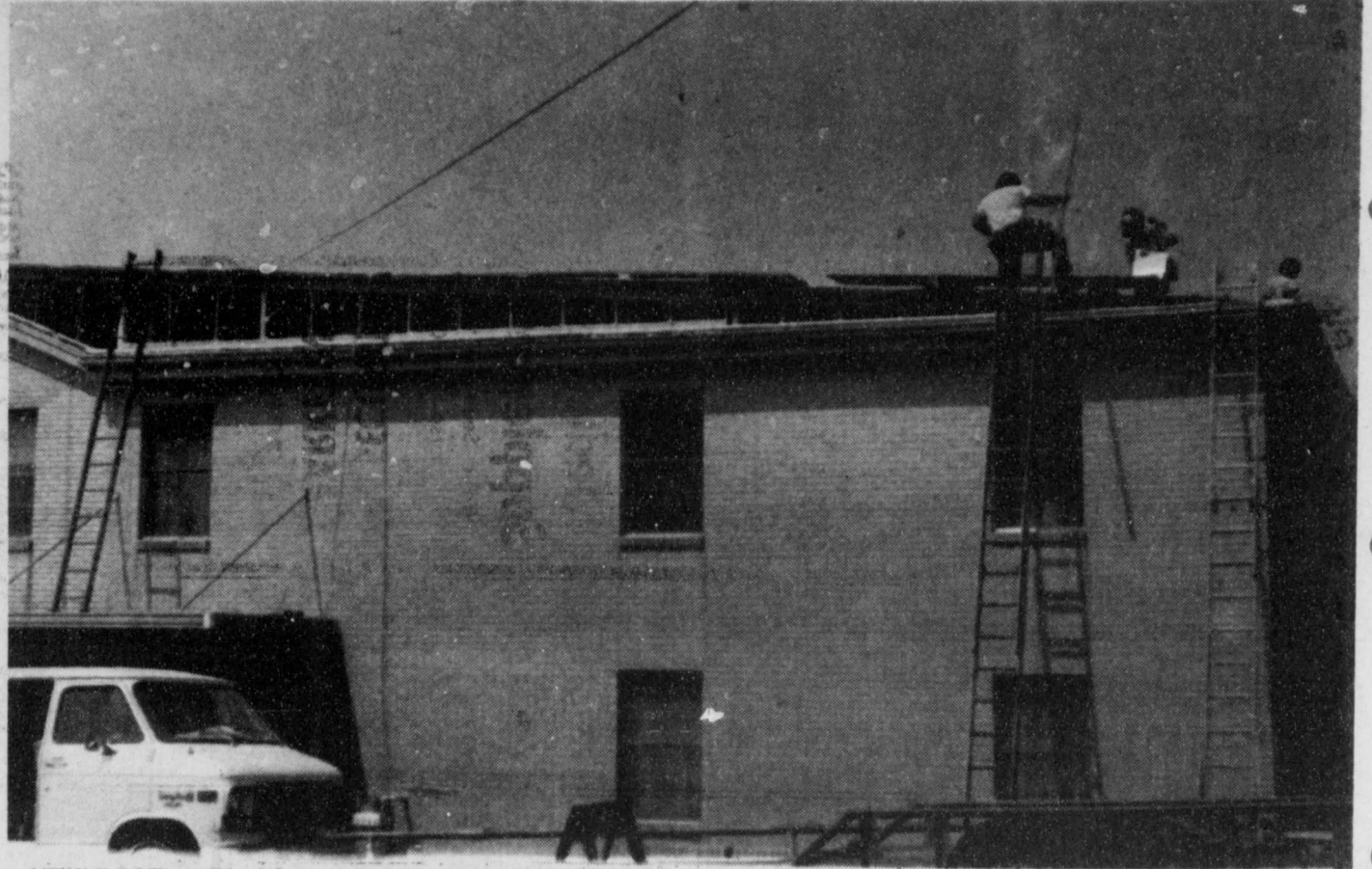
NEW ROOF—The First Baptist Church of Bogata is receiving a new roof at present. The old, flat,
