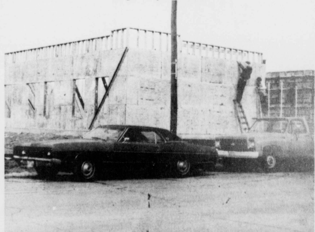
GOING UP FAST—Once the weather finally let construction workers pour the slab, the Talco
