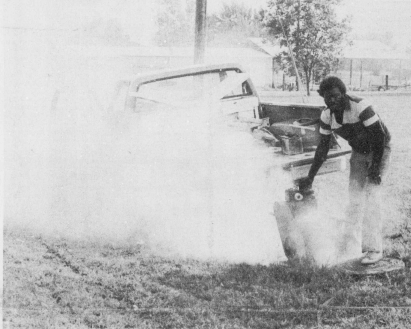
SMOKING—smoking of sewer lines in the city of Bogata began Monday. The lines are being tested for leaks or defects. The smoke is harmless, but abundant. (Staff Photo by Linda Tabb)
