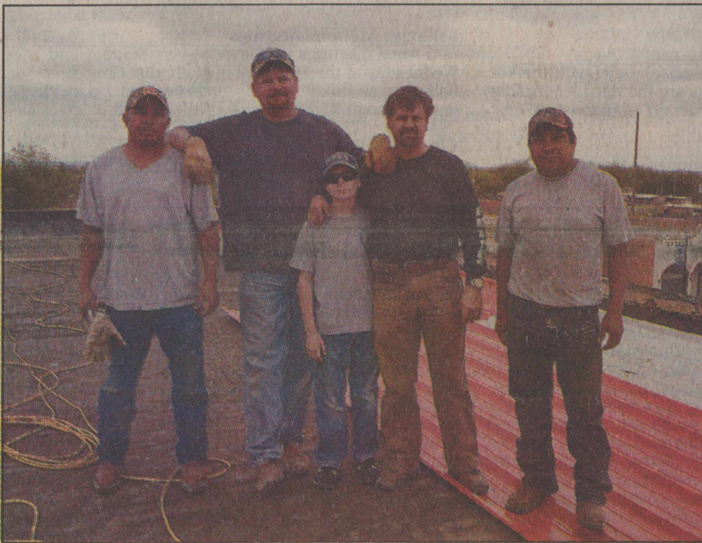
PHOTO: RUBEN CANTU-RODRIGUEZ Roofing crew members working at the Paladín Community Services building are left to right: Facundo Castillo, Jason Boatman, Cody Johnson, Nathan Johnson, Emilio Castillo.
