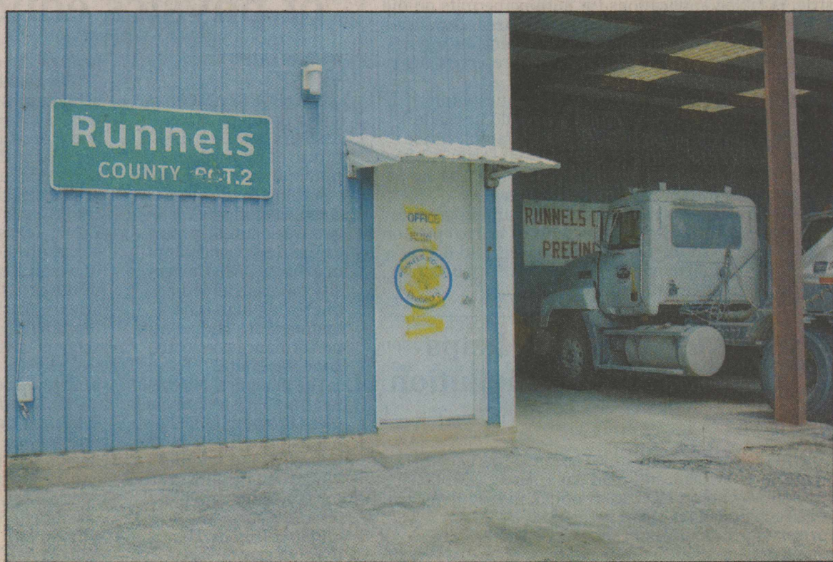
PHOTOS: RUBEN CANTU-RODRIGUEZ The building, equipment and vehicles in the Precinct 2 County Barn, in Winters, were spray painted on Thursday. Over the weekend the window of a backhoe was also shot at and destroyed.
