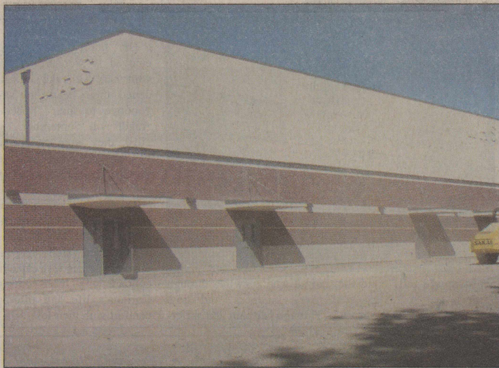
LAST WEEK the construction crews were preparing to pave the surrounding area of the new gymnasium. Photos: Ruben Cantu-Rodriguez
