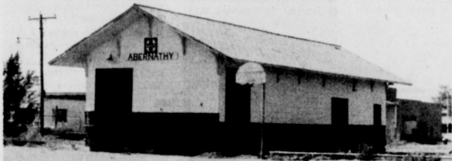
DEPOT MOVED TO NEW LOCATION...and remodeling will begin soon on the inside to convert the building into a Senior Citizens Center for Abernathy. (Review Photo)
