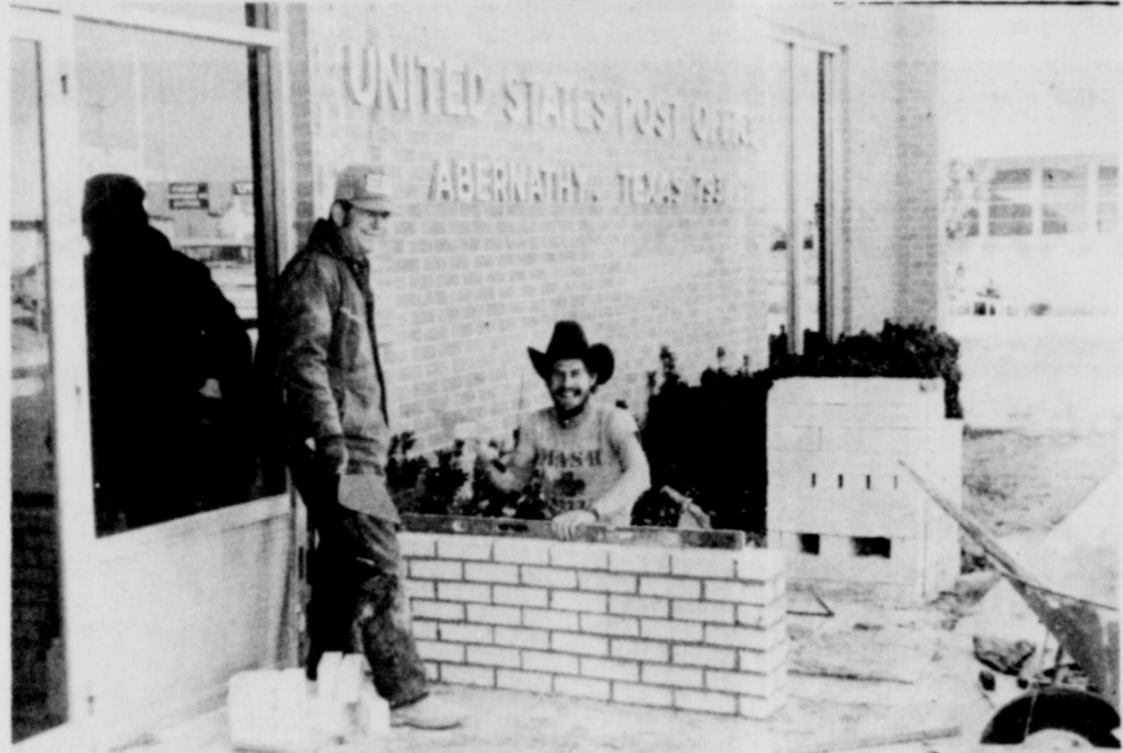
REBUILDING THE POST OFFICE WINDBREAK is Rev. Tommie Beck and son Mark. Tommie used to be a brick layer, and Mark is presently a brick layer. The wall is designed to shield the wind off the front door and the two outside drop boxes. (Review Photo)
