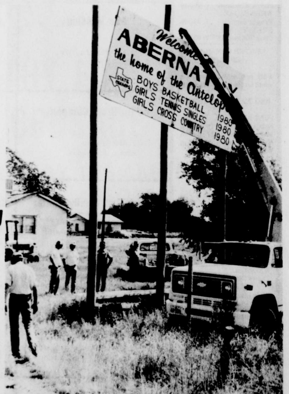
CHARLES BOWEN, accompanied by several local men, make an attempt to put the Abernathy Antelope welcome sign up on the south side of town. The signs had been lying on the ground for over a year and showed signs of aging. They had to be cleaned and the rotting wood reinforced with 2x6" 16 ft. boards. (Review Photo)
