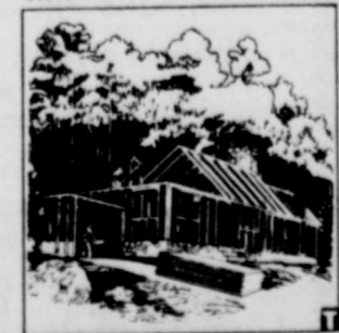
WOOD'S FLEXIBILITY AND STRENGTH make it an excellent construction material.
