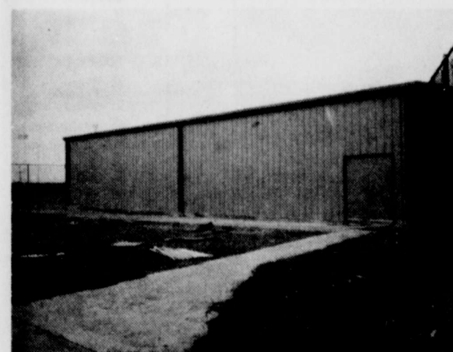
New Elementary School P. E. Class Building.
