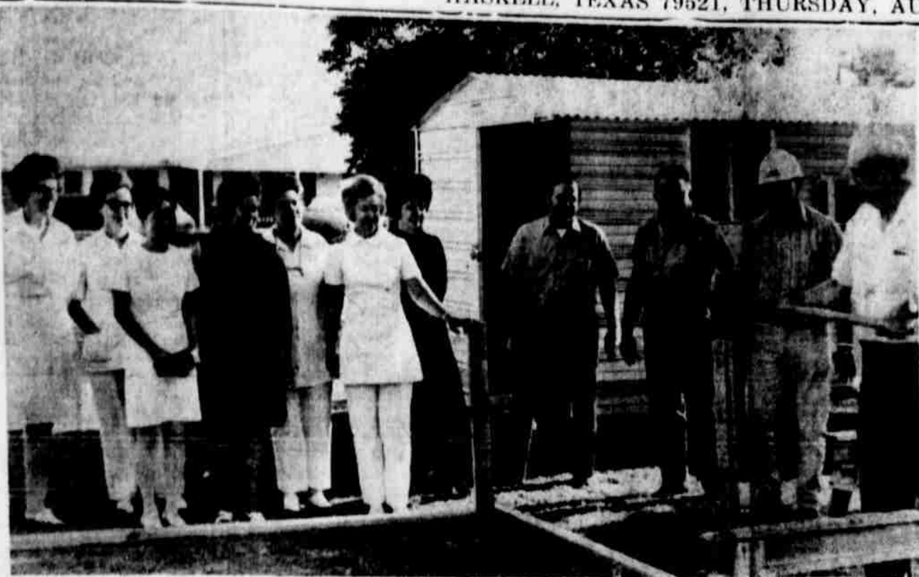
DRIVING THE FIRST STAKE and officially opening construction of the addition to the Haskell Memorial Hospital is Administrator Alfred Turnbow (right). Observing the event from a safe distance are: (l. to r.) Inez Gholson, Jean Love, Jong (Kim) Suk Koo, Mildred Berry, Ruth Ezill, Ruby Martin, Beverly Philpot and Jerry Weatherly, all members of the staff at the hospital. A.E. Donaldson and L. C. Saylor, both of Fort Worth, represent the firm of Haws and Garrett Construction Co., which is in charge of the construction project. (Staff Photo)
