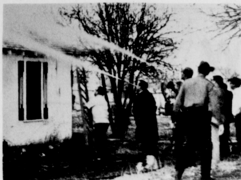
ABERNATHY VOLUNTEER Firemen are shown here fighting a house fire. Used for storage, the house is next door south of Davis Grocery. It was badly damaged. (Photo by Virgil Wade, Abernathy photographer)
