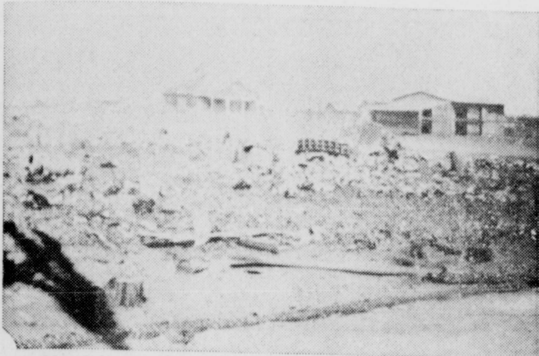
THIS IS the ruins of a store and the Abernathy post office, which burned in about 1920. J. C. Arnett was postmaster at the time, and the post office was in Bud Pipkin's store. It was located on the west side of what is now Avenue D, somewhere between the bank and Richter Insurance office. House in the background is the one now occupied by Chambers Funeral Home on Avenue E at 10th Street.
