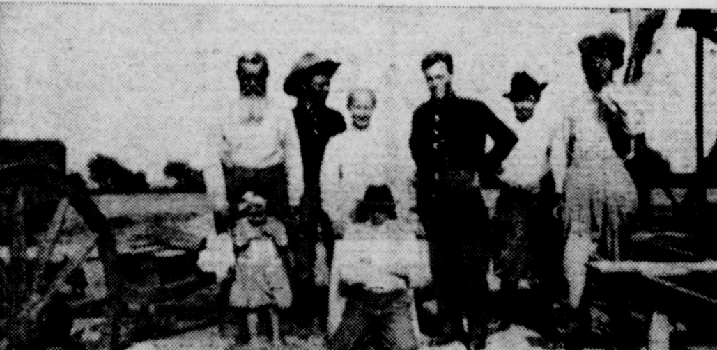
This picture of the entire family, made at the time of making an addition to the old homestead place, about 1909, from left to right, Dr. Harp, sister Pauline, Walter Harp, Mother Harp, Earlington kneeling, Robert, and Edgar, and the carpenter who had charge of the construction.
