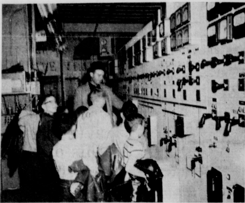
WILLIE FLORENCE, Tuco Power Plant manager, is pictured above showing a group of Abernathy 4-H Club members the electrical control panel in the "control room" at the Tuco plant. At the time the photo was made, Florence was showing the boys the control switch that operates the oil circuit breaker through which power is furnished to the Abernathy line.—(Rev-Foto).
