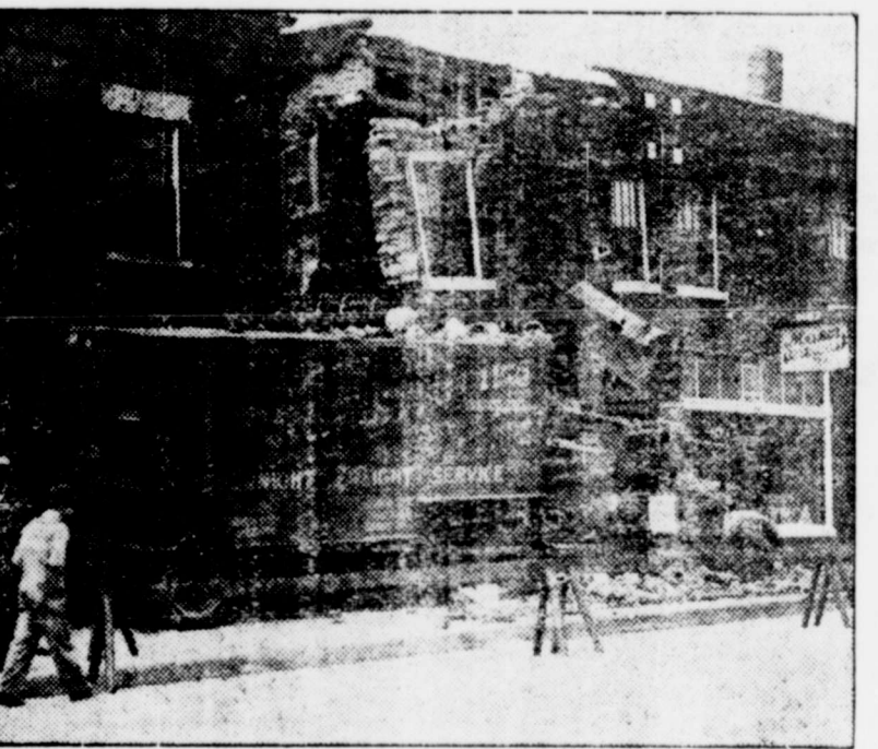
Kansas City, Kans.—A 15-ton truck on a wild rampage finally came to a stop at this hardware store. A part of the damaged wall of the building rests on the truck, which cannot be removed until workmen brace the structure so that wall will not collapse. Such destruction of property, particularly by irresponsible itinerant truckers, is the reason why safety councils nationwide are seeking more stringent laws thoroughly regulating motor transports.
