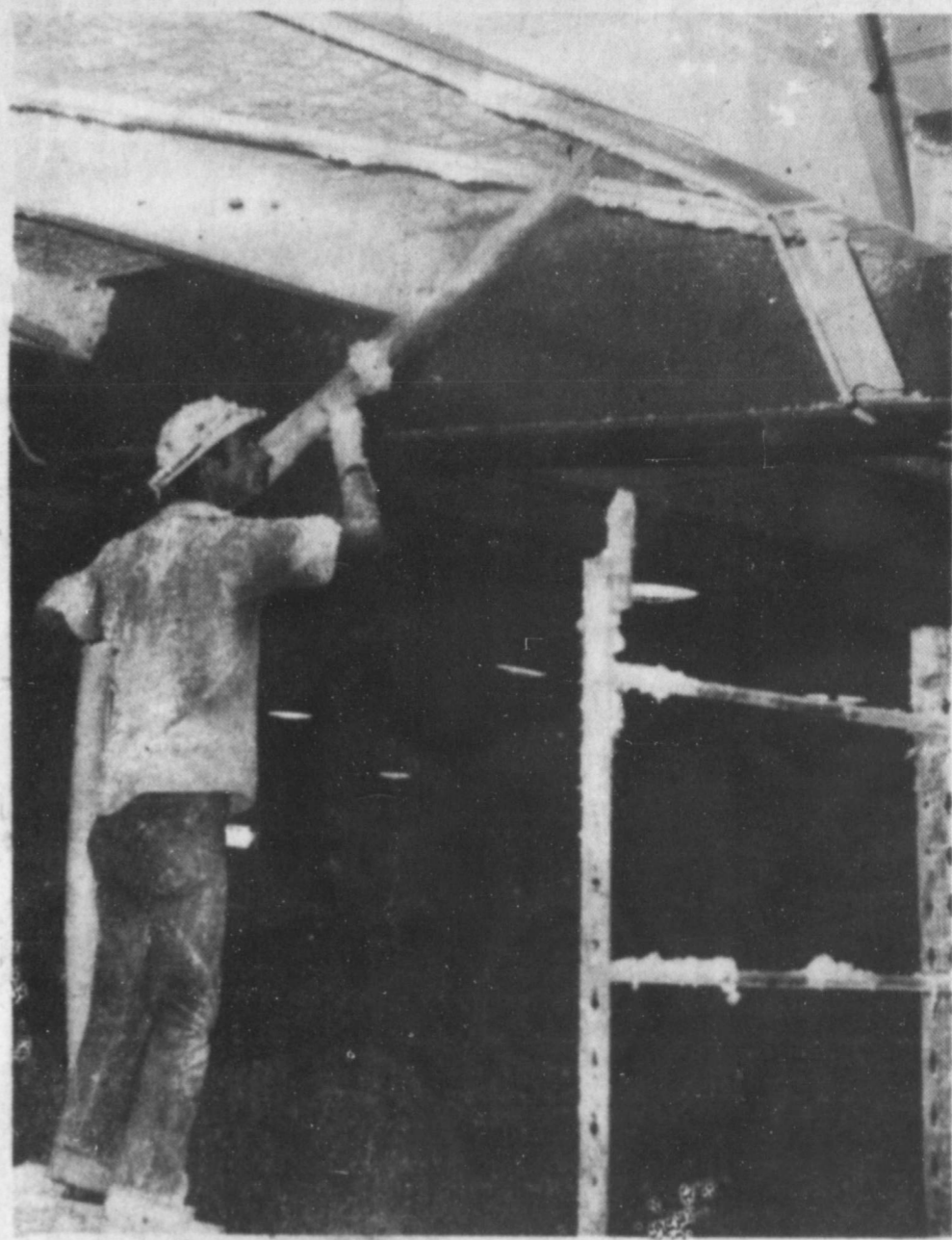
ROOF REPAIR JOB AT THE JAYTON HIGH SCHOOL
