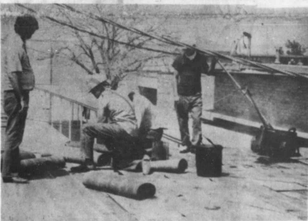
WORKMEN PUTTING ON A NEW ROOF AT THE SCHOOL
