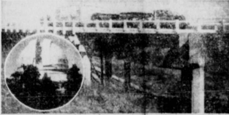
TRAILER CRADLES GIANT MIRROR. The world's most fragile load, the 200-inch Falomar telescope mirror, valued at $400,000, is carefully transported by truck-trailer on a 160-mile trip from the California Institute of Technology to the Palomar Observatory atop Mt. Palomar (inset). The mirror was packed in a special shockproof case and loaded on a 16-wheel Fruehauf Trailer. Combined weight of the mirror, case, truck and trailer was 60 tons.
