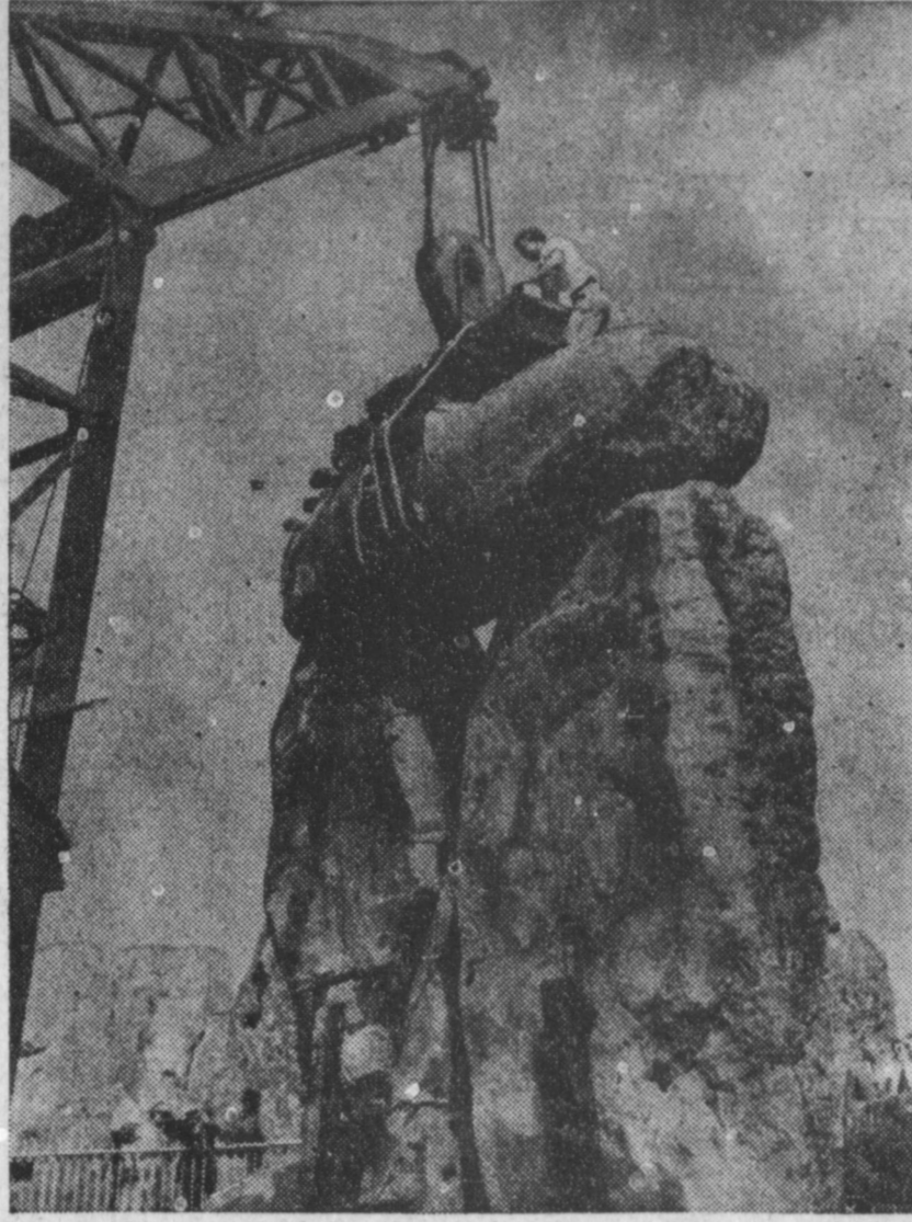
STONEHENGE RECONSTRUCTED—A giant lintel is lifted into place atop the Druid's Circle in Stonehenge, England. The Circle, popularly supposed to have been the worshipping place of the ancient Druids, is being reconstructed as a monument.
