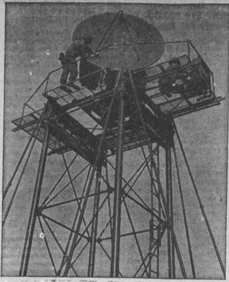
PORTABLE STORM RADAR —Two Signal Corps soldiers finish assembling the Army's new weather eye for spotting significant storms at distances of 200 miles. The 25-foot tower can be set up in a day to allow Army scientists to predict within minutes when a storm will strike any spot within range.
