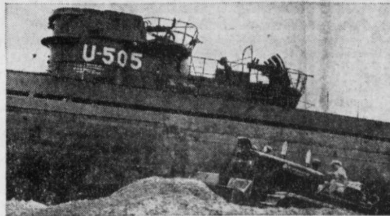
When breakers threatened to wash away cribbing supporting beached sub, International TD-24 crawler tractor was brought in, bladed sand into nine-foot-high protective dike.
