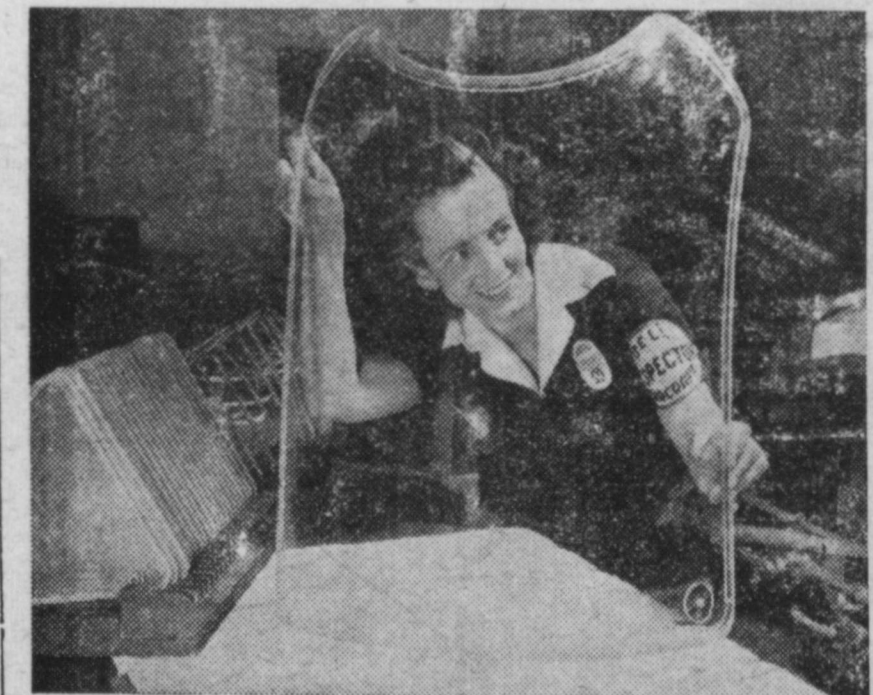
One of the many women workers at Bell Aircraft's Buffalo plants inspects a sheet of molded plastic before it goes to the assembly line for installation in an Army fighter.
