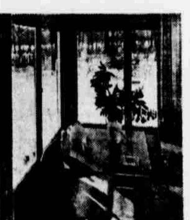
The variety of quality wood window styles makes it easy to choose the right one for each room. Ponderosa pine slider units were used in this corner to allow wide visibility and easy operation.
