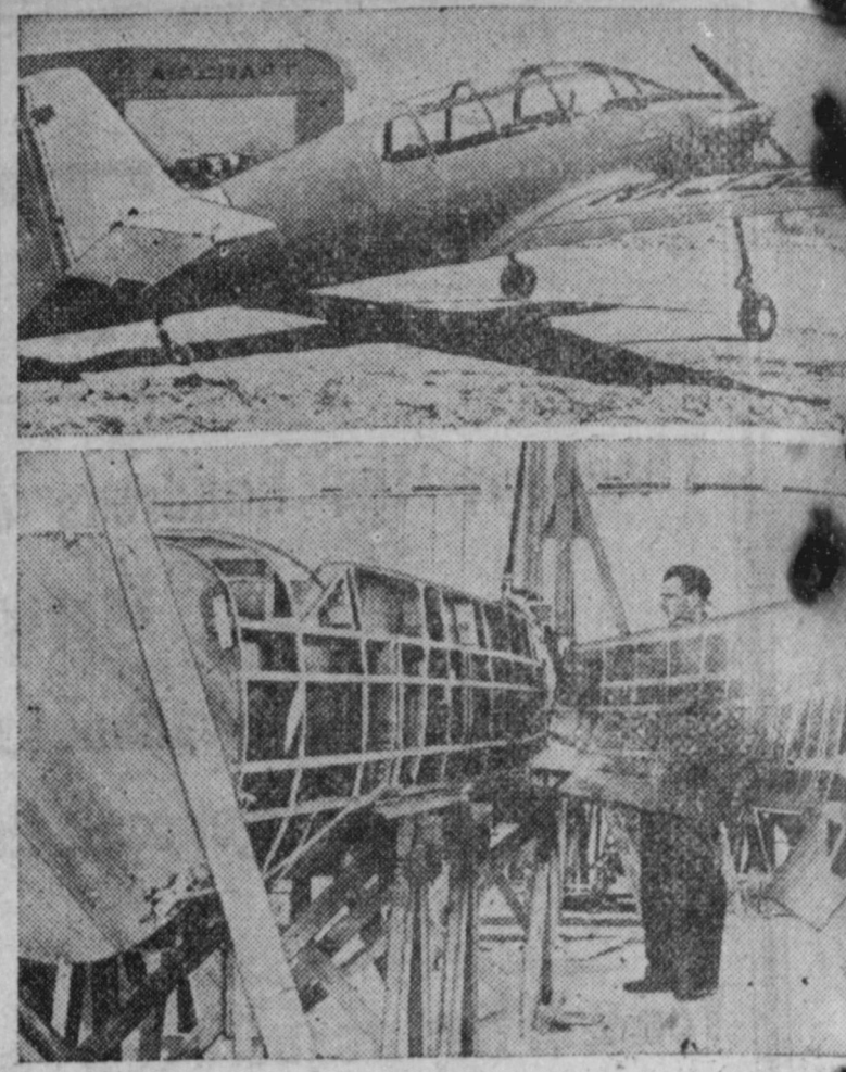
In order to solve the metal shortage in plane production, piano and furniture men have built a plane made 90 per cent of wood. Fleets of these huge wooden troop-planes, capable of carrying men and munitions at 200 miles per hour, are nearing reality. Below you see these experts making the plywood sides. On top is the completed plane.
