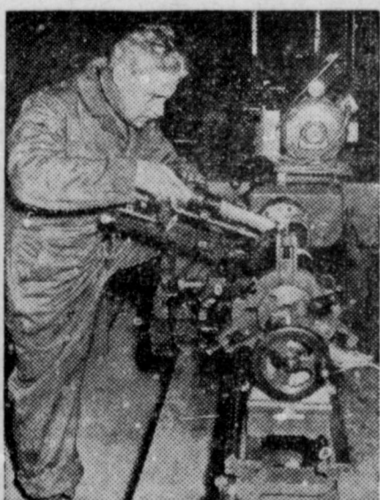
Working on a small crankshaft grinder adapted to a lathe is Colonel Stilwell of Camp Shelby, Miss. The colonel expects to put the knowledge gained at this school to a test in the near future.
