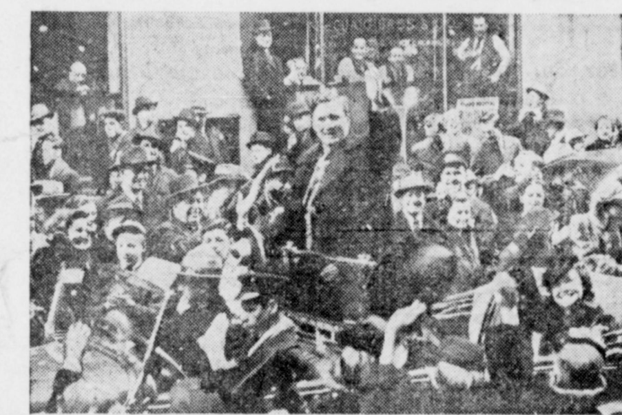
As great an ovation as any which he received when running for the presidency was tendered Wendell L. Willkie when he visited Montreal, Canada. St. James street forgot to be staid when he and Mrs. Willkie drove down its length to a civic welcome at the city hall. They are shown waving as they passed the Canadian Bank of Commerce.
