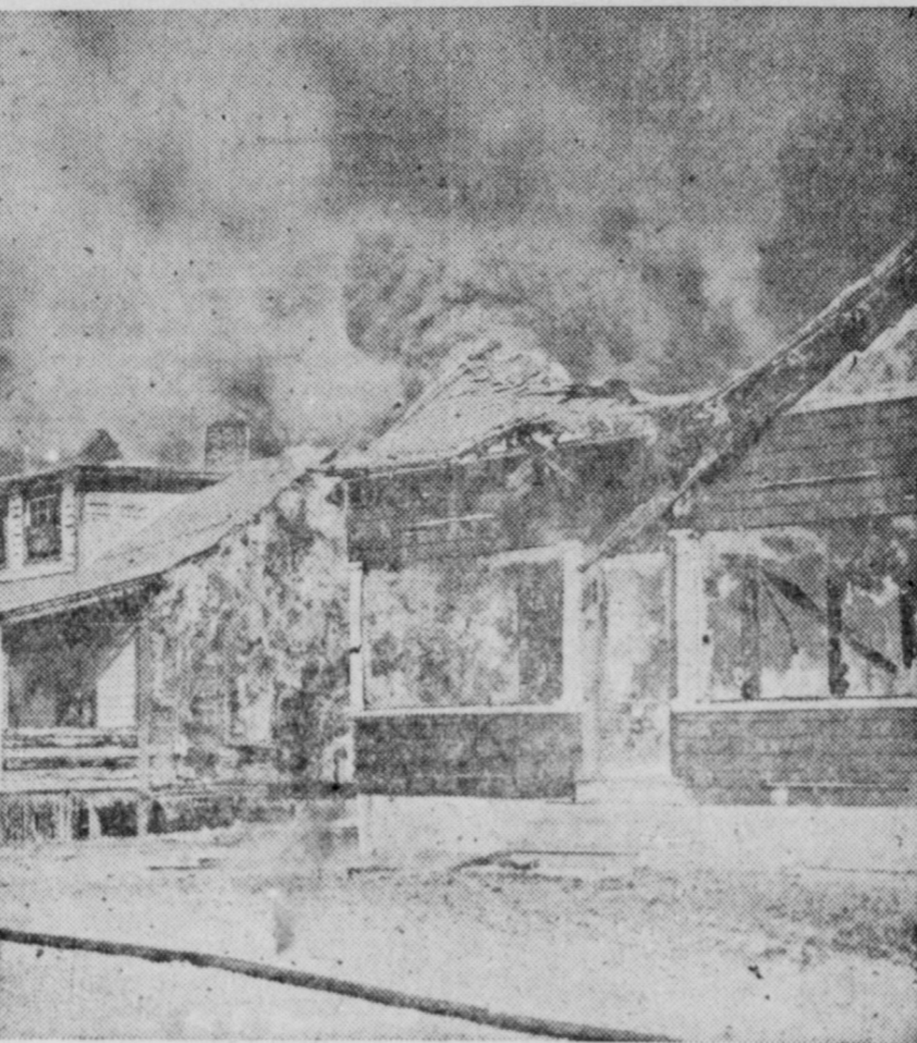
Damage estimated at about $2,000,000 was caused in the Ocean Bluffs, Mass., area as the result of a fire that destroyed a church and leveled more than 450 cottages. Only a timely shift in wind saved hundreds of other houses. The above photo shows a row of cottages burning fiercely when the fire was at its height.
