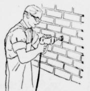
Portable drill fitted with wire brush cleans masonry quickly.
