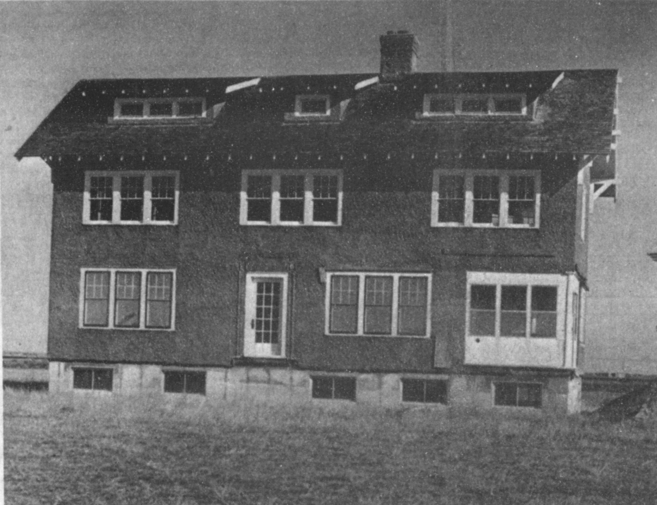
JANES RANCH HOUSE LOOKING BETTER --Re-roofing, new windows, paint, a foundation and other renovations are making the former Janes Ranch House, which was formerly located east of Muleshoe, look a lot better. The building will be turned into a historical museum when the renovations are completed. It is located at the Ranching Heritage Center.
