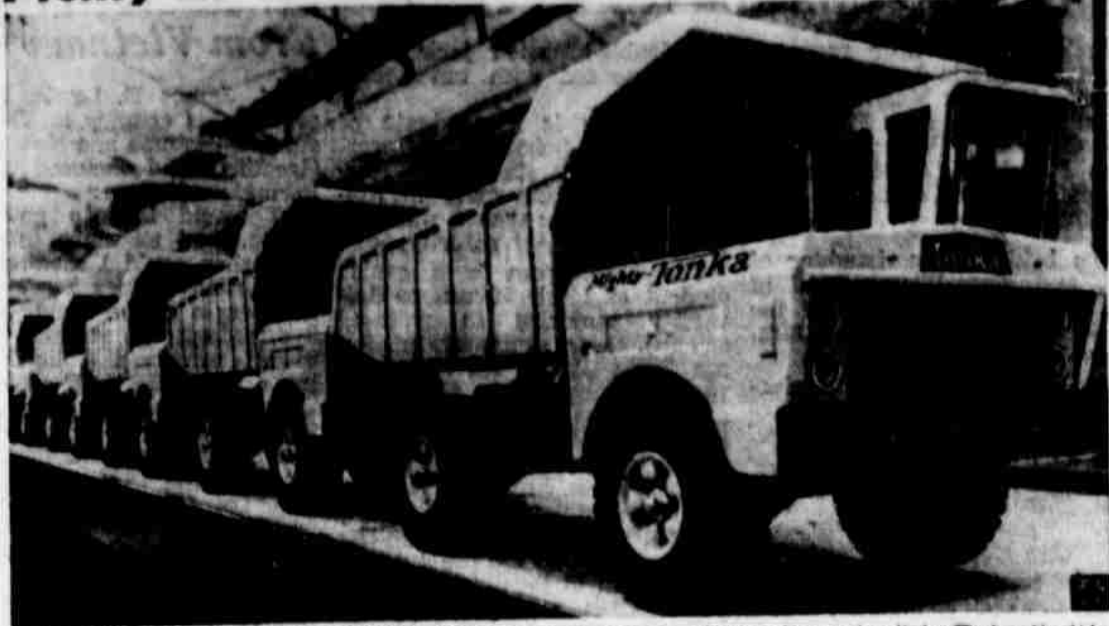
THE WORLD'S BUSIEST TRUCK assembly line, shown here, isn't in Detroit; it's in Mound, Minnesota, where Tonka Corporation is producing tens of thousands of steel toy trucks every day to meet its 1967 goal of more than ten million individual toys before Christmas. Rolling off automotive-type assembly lines, these dump trucks are made of automobile-gauge steel, finished with real truck paint.
