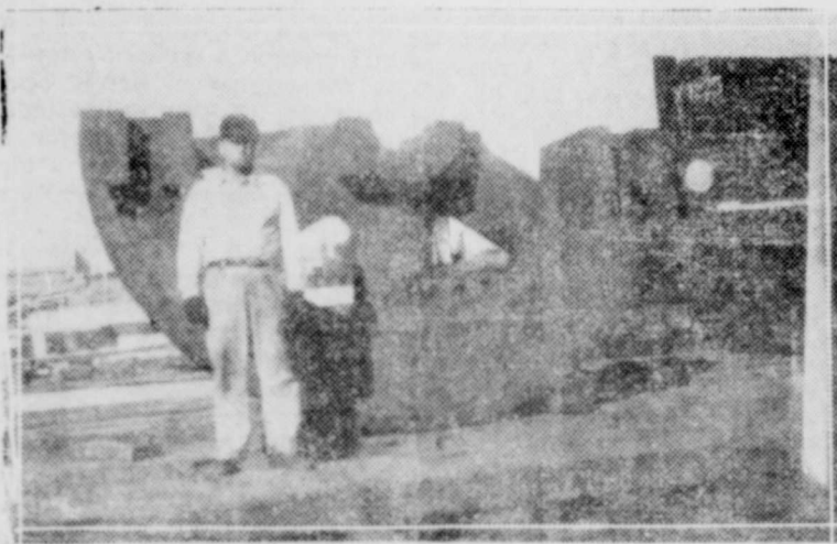
The half of the huge wheels that are being used at the plant. Each wheel on the two machines weighed 84,000 pounds. They are the heaviest that are used in any structure anywhere. Dewey Farar is standing by the wee 42,000 pound half.
