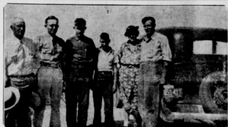
O. J. Addis and family of Toulon, Illinois were the first to cross the reconstructed gap at the Red River Bridge. In the picture are: T. M. Motz, state engineer, W. C. Peterson, federal engineer, John and Robert Addis, Mr. and Mrs. Addis.
