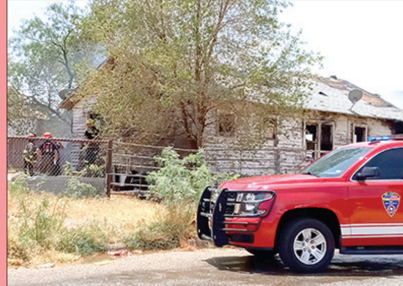
Big Spring firefighters, left, examine the wreckage of a structure fire which burned Thursday afternoon at the intersection of 18th Street.
